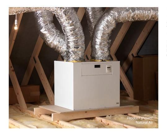
Mechanical Ventilation and Heat Recovery (MVHR) is a solution that creates air flow within buildings, where natural ventilation is limited.
