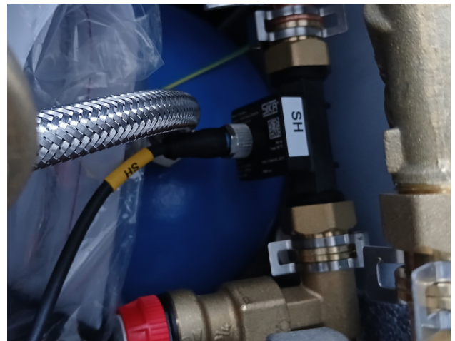
Fig. 72 : Remove SH Flowmeter Cable
