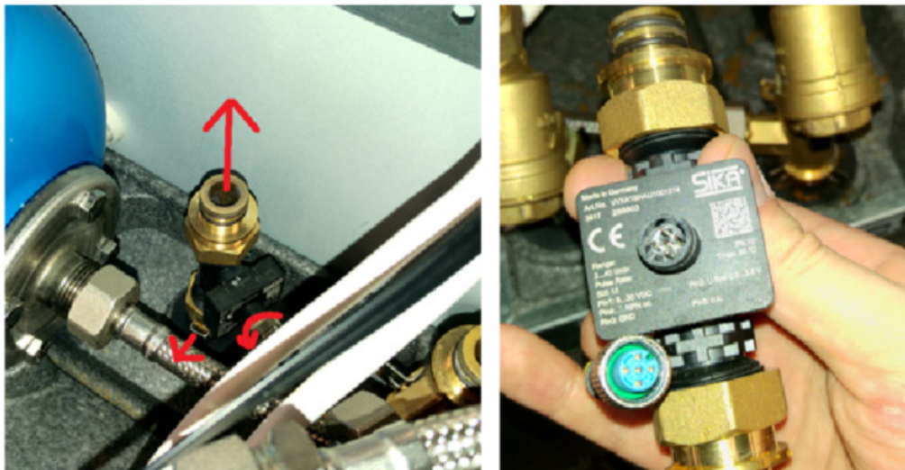
Fig. 99 : Replacing the flow meter
