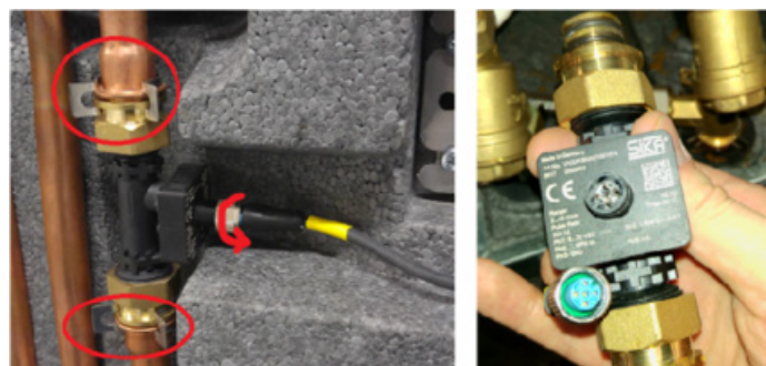
Fig. 102 : Flow meter removal
